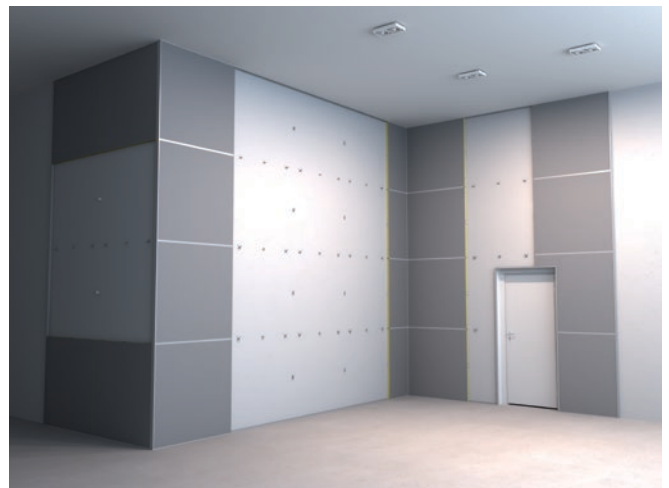
3.10 Cover all remaining horizontal joints between panels by clicking T24 profiles into the T fixing brackets. Horizontal profiles should be cut to an exact dimension of M-12 mm. Ensure the outer ends of the horizontal tees are covered by the J-channels.
