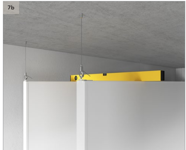
Place a level on top or underneath the baffles to ensure their evenness. Levelling can be done by releasing the lock on the hook and pulling on the wire rope.
