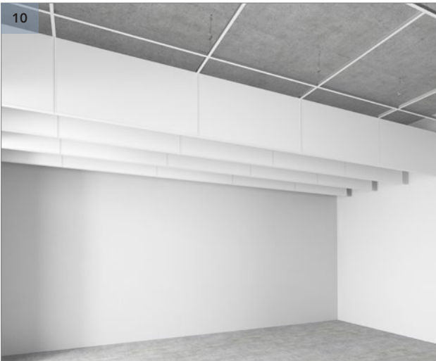
Fix the remaining Rockfon Universal Baffles to the T24 grid and align them using the dimples on the end of the baffles.
