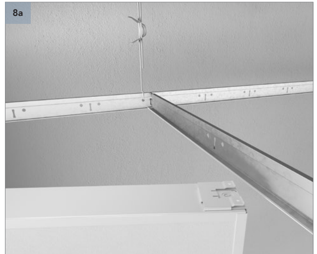
Fix the Rockfon Universal Baffle to the suspended Chicago Metallic T24 grid.
