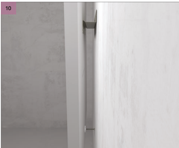
Place your Rockfon Eclipse Wall panel on the wall fixing profile and adjust the distance holder until the Rockfon Eclipse Wall panel is level. See 10 - Detail.
