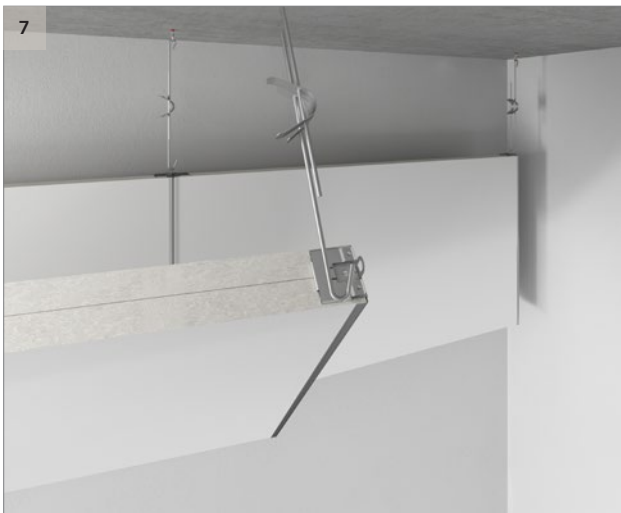
When necessary, twist the baffle to secure the eyelet onto your quick-hangers.
