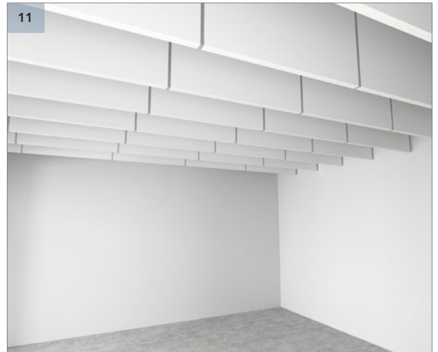
Fix all the remaining Rockfon Industrial Baffles in the room.
