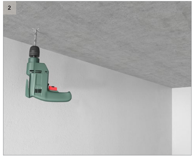
Drill where you have marked drilling points.
