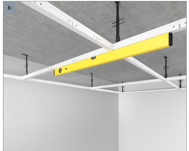
Install T24 ECR cross tees to main runners every 1200 mm. Ensure the grid is leveled before installing the baffles. Use the locking pins to adjust right level for all T24 profiles. Note: if the T24 ECR grid is not level, the baffles are not level either!
